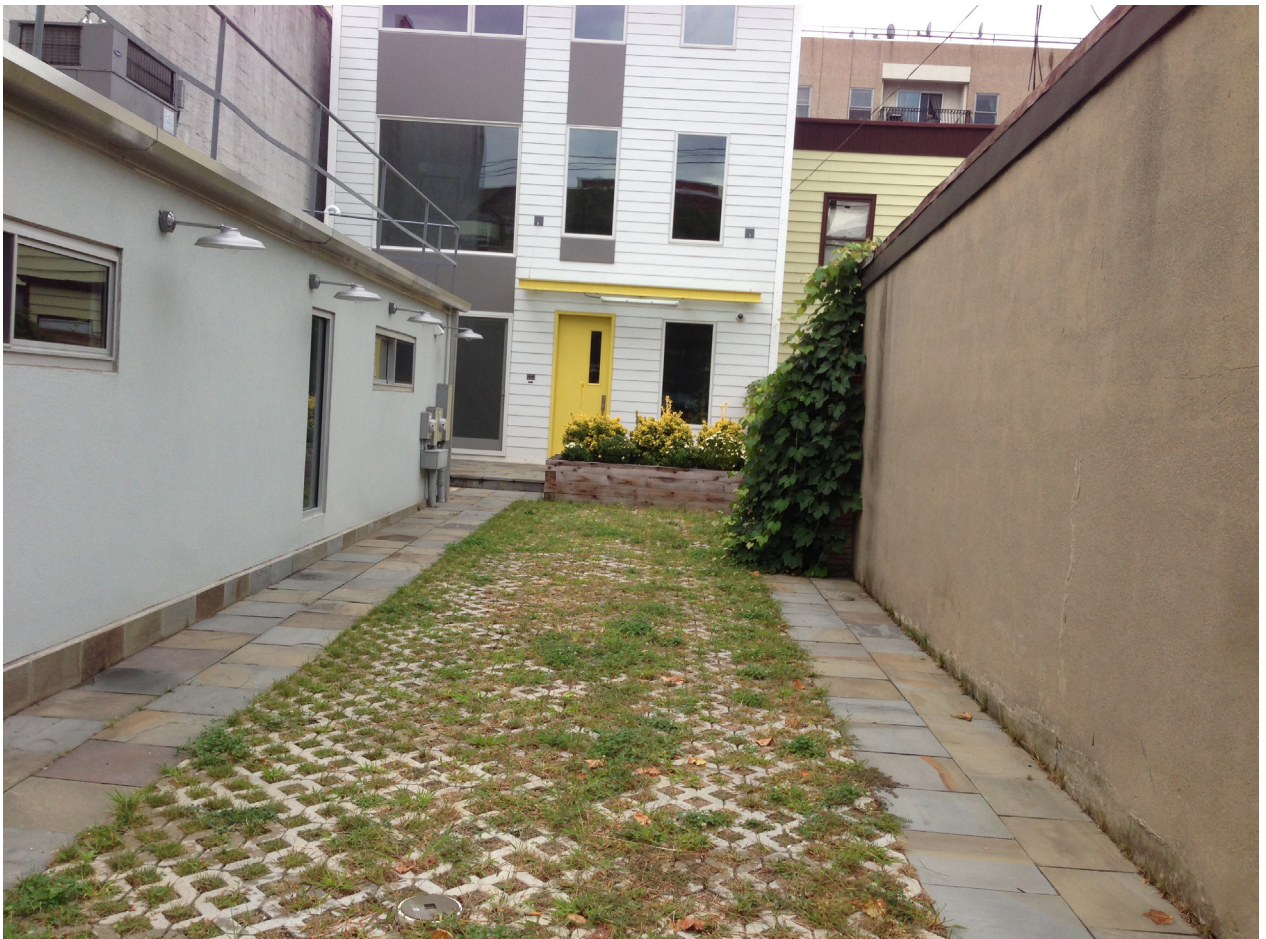
Permeable paving at a recently constructed house in the study area
